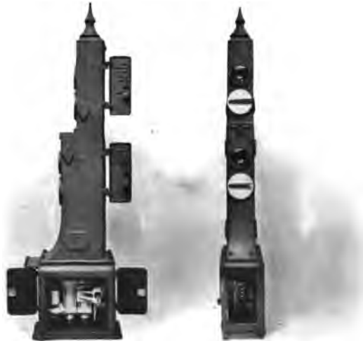
Electro-Pneumatic Block Signals, New York Subway
